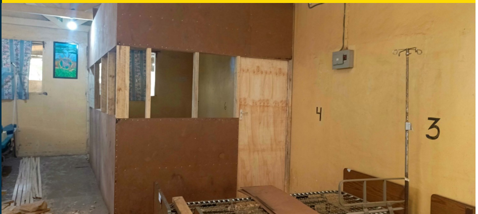
Small Neonatal unit in early stage of construction.
